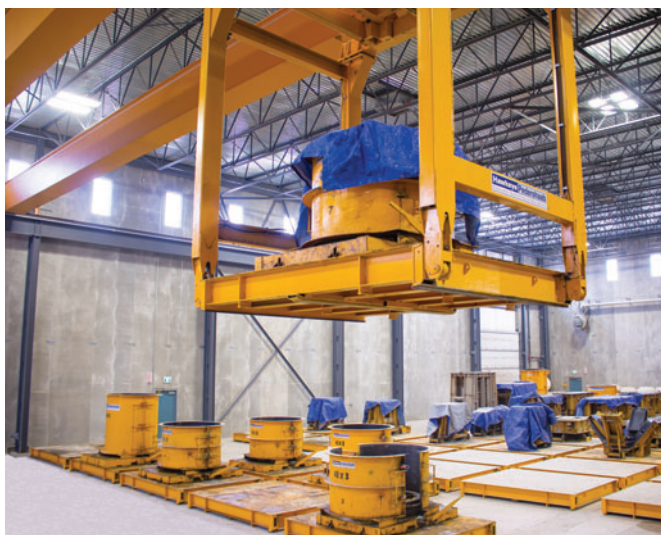
Inventory is automatically handled by an overhead manipulator.
