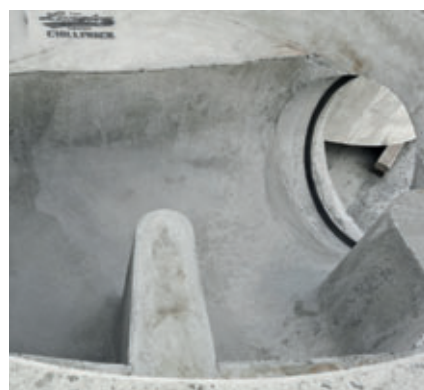
Problem solved – two small pipes instead of one large one.
