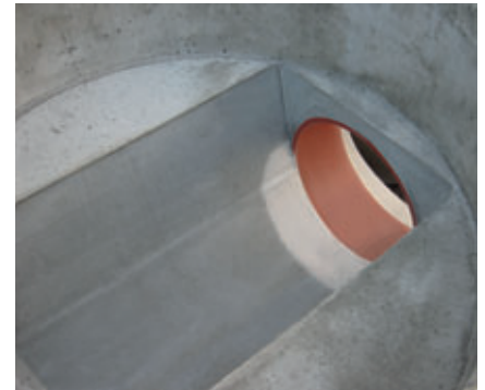
Tubobel often has to connect special pipes with large connecting pieces.
