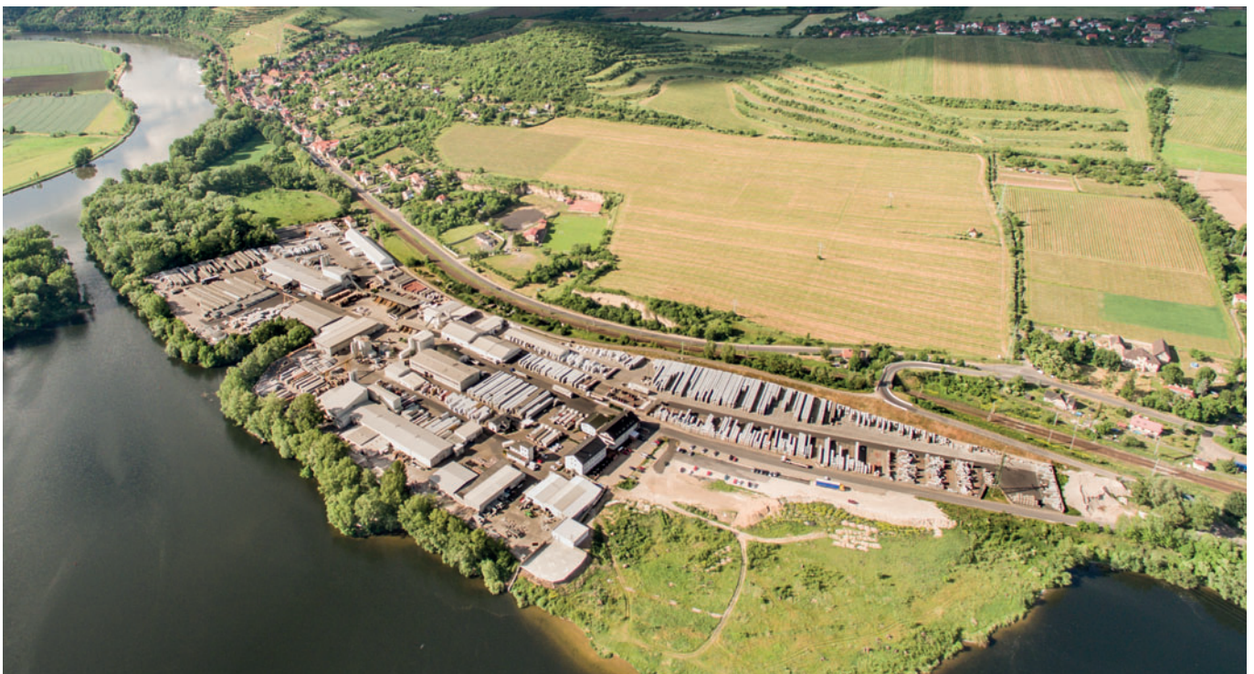
The CS-Beton plant in Litoměřice
