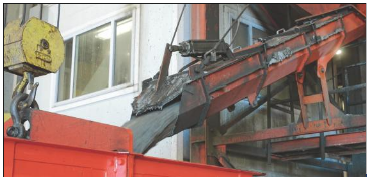
Charging the Crete Hawg
