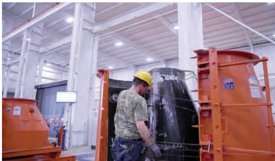
Each form contains an RFID tag that contains pertinent information like location, processing times, concrete mix, vibrator settings, among others.
