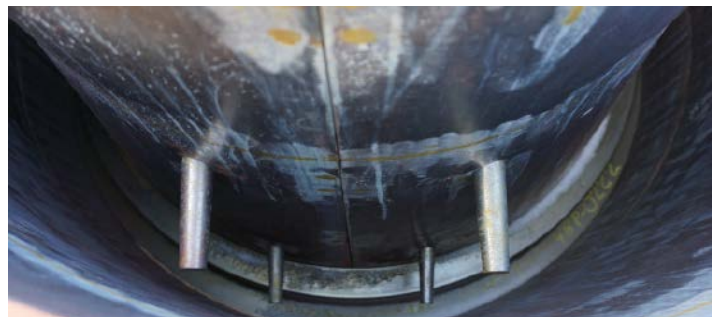
Manual Step Pin Assemblies or Cast-in Plastic Break-off Step Inserts. Several make/models to choose from.
