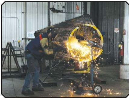
Prefabricated Flared End Cage
