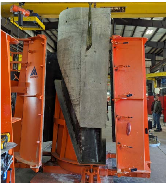
3. Using the added SmartConnect® to engage the hydraulic strip assist cylinders; break the bond of the concrete to the inner core.
