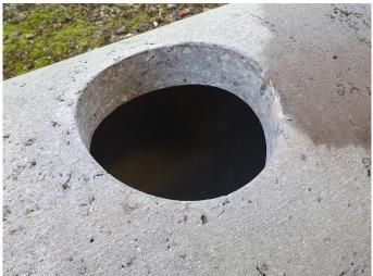
1. Core a 178mm (7") diameter hole in the concrete pipe. Ensure it is perpendicular.
