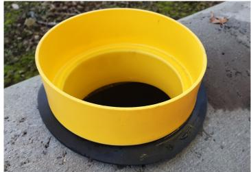
**4.** Ensure the socket is pushed fully home, fit the second seal.
