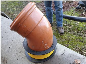
**5.** Ensure the pipe has a good chamfer, lubricate the inside of seal and the spigot on the pipe and press into the seal. Ensure the pipe is fully engaged.
