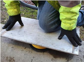
3. Lubricate the inside of seal and the spigot on the branch adaptor with a high quality lubricant. Push the branch adaptor into the seal. Using a board can help maintian alignment and make assembly easier.
