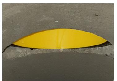
**6.** Neither branch adaptor or pipe can protrude into the flow of the pipe.
