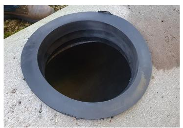
2. Ensure the hole is clean and free from score marks, a poor quality hole may reduce the effectiveness of the seal. Push seal ST100 into the cored hole, no lubricant is required.
