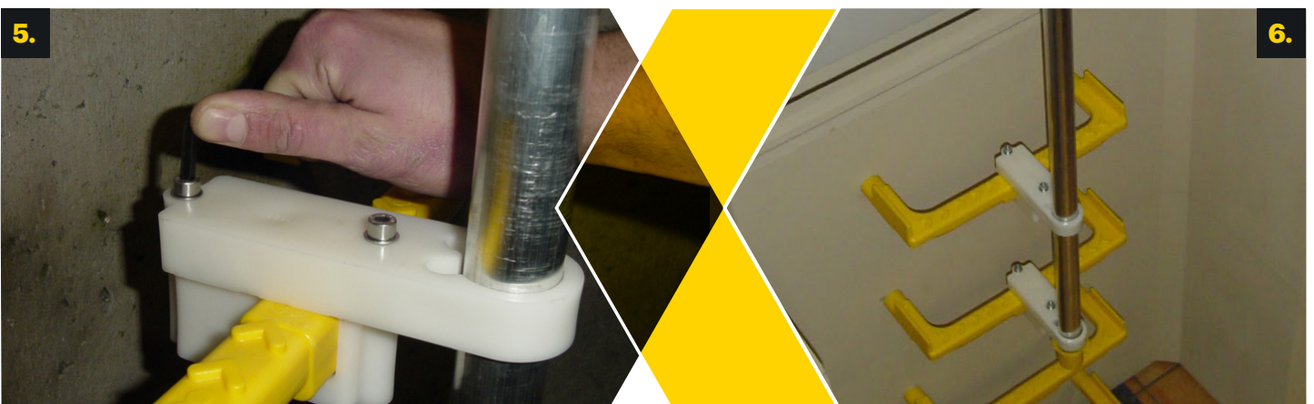
5. Tighten 4 screws with 5mm Allen key.
