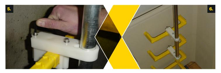
Tighten 4 screws with 5mm Allen key.
