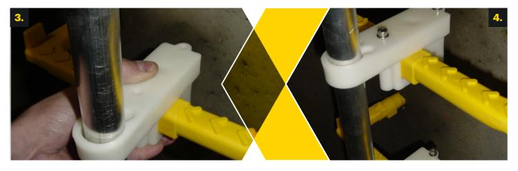
Fit upper half of bracket ensuring correct fit with step and lower half of bracket.
