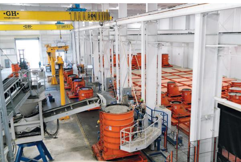
Specialized workstations on the Prima at Tindall Infrastructure in Spartanburg, SC.
