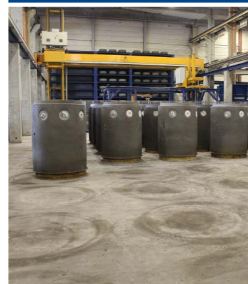
Open floor curing of sand traps
