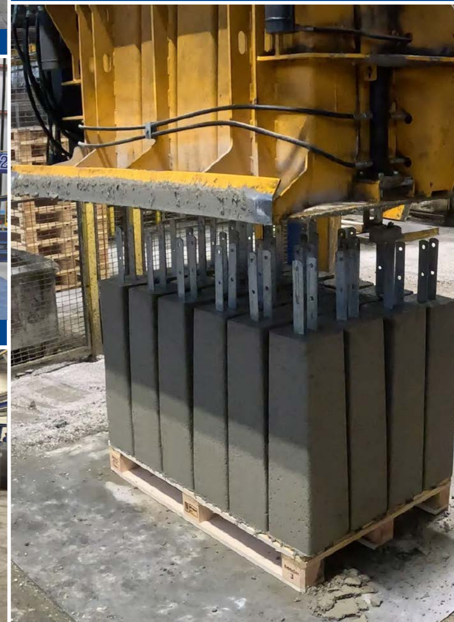
Concrete post demolding
