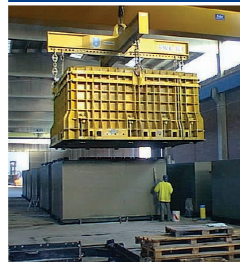
Demolding of box culvert
