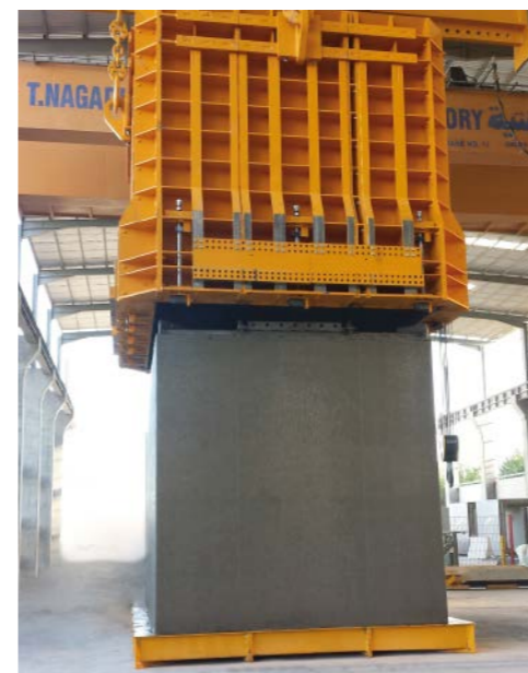
Demolding of box culvert
