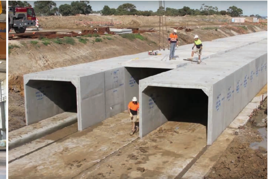
Box culvert installation
