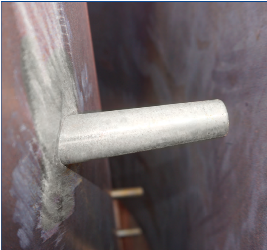
Blockout Step Pin/Hole Former
